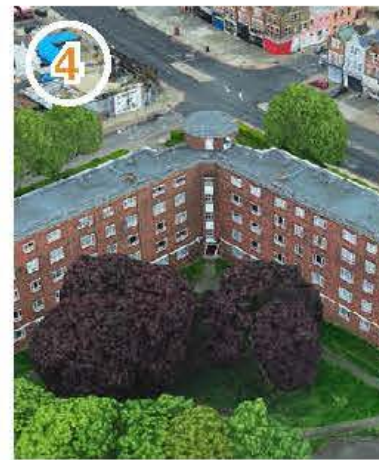
Randisbourne Gardens 5 storey
