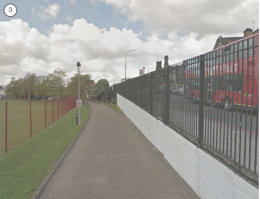
VIEW LOOKING WEST ALONG THE A205 TOWARDS THE BRIDGE
