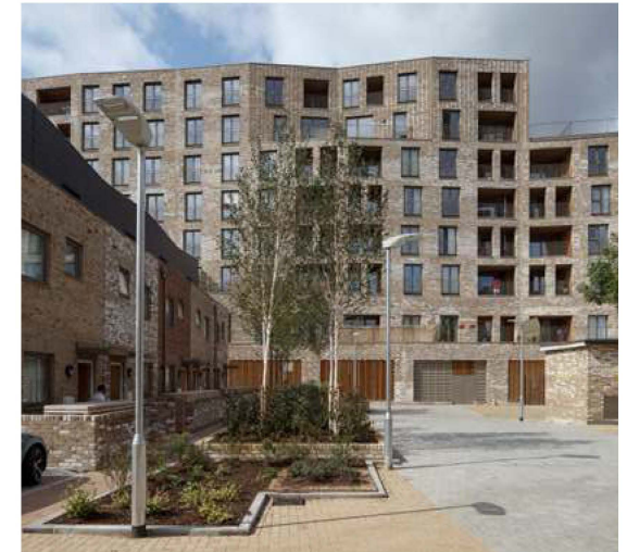
Fig. 9 Residential led development where by tall block facing the main road encloses lower density terrace at Prowse Court and Lord Graham Mews, London N18 2FF
